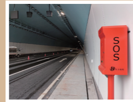
Highway tunnel in Chongqing, Gaoteng
